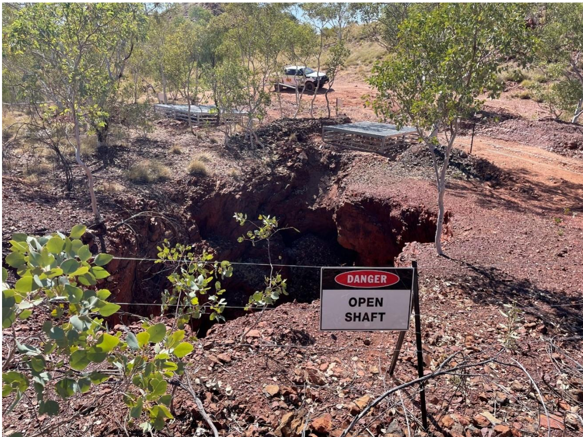
Image: Safety works near Tennant Creek
