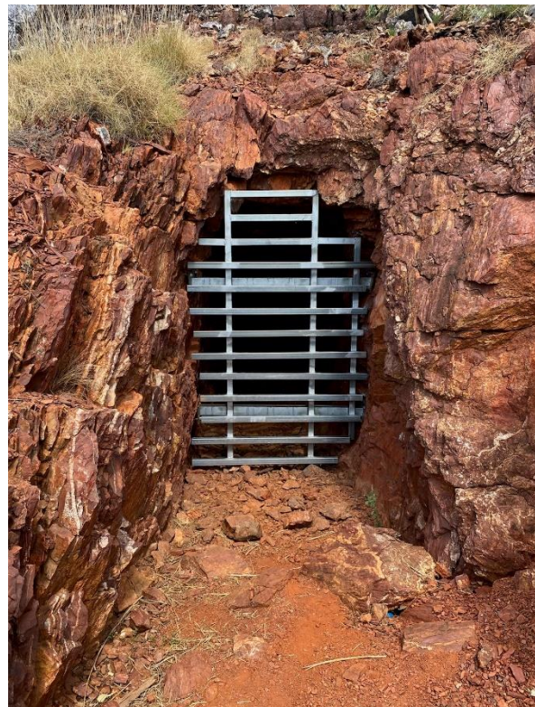
Image: Grate installed at Queen of Sheeba
