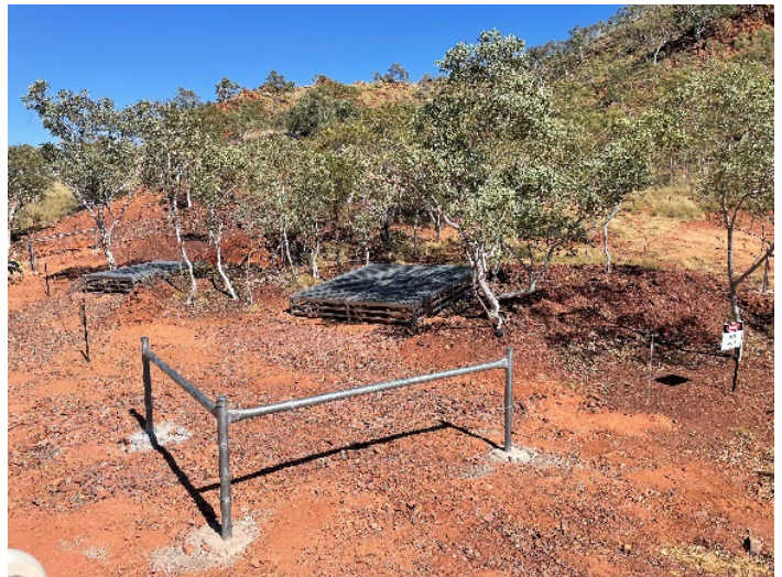
Combination of Controls: grates, fencing and signage
