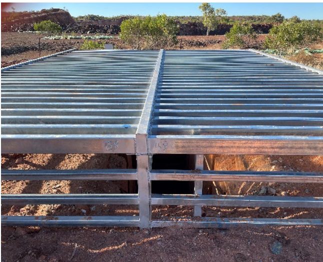
Grates enabling wildlife access
