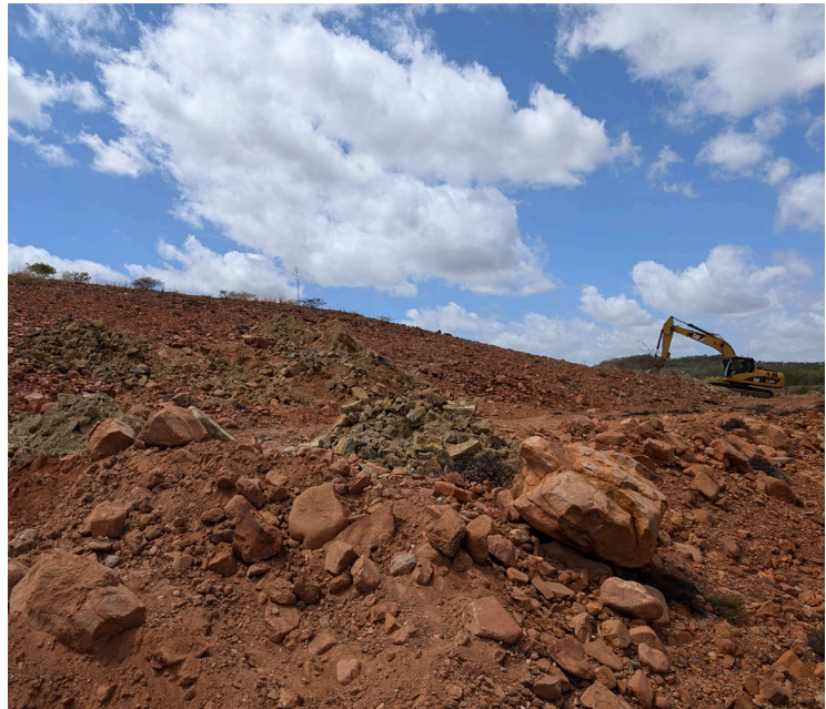
Test pitting works associated with mine waste characterisation
