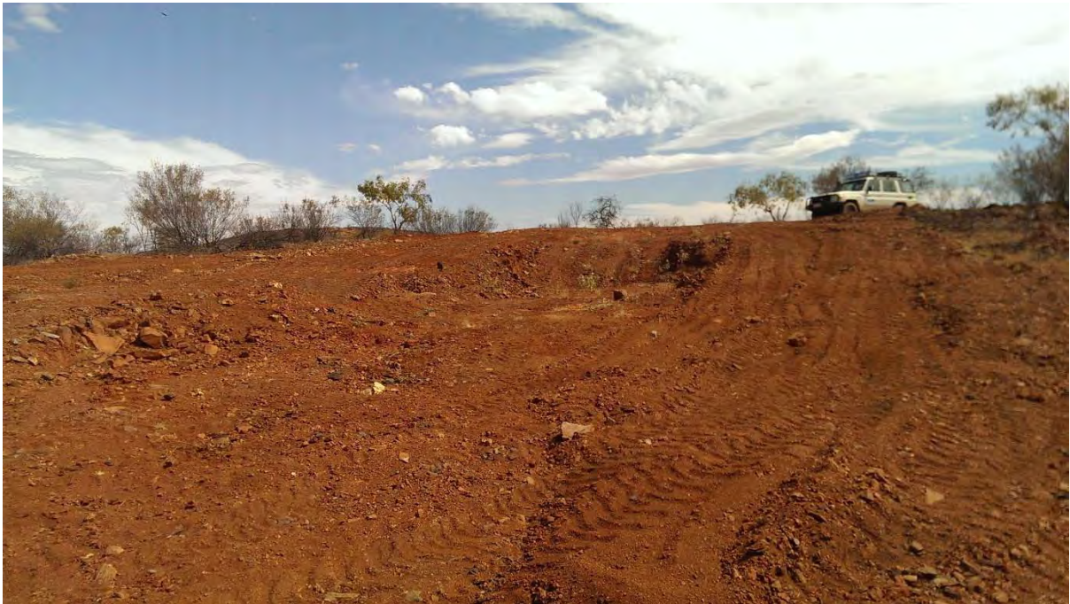
Figure 1. BYD001 under rehabilitation
