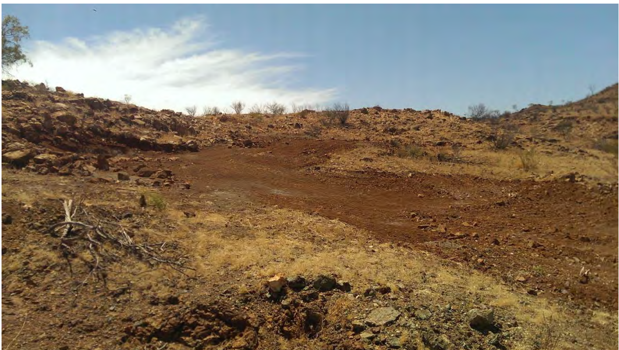
Figure 2. BYRC003 under rehabilitation
