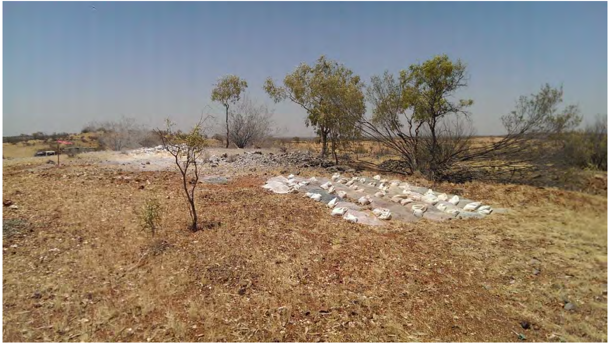
Figure 24. GHRC002 – rehab required
