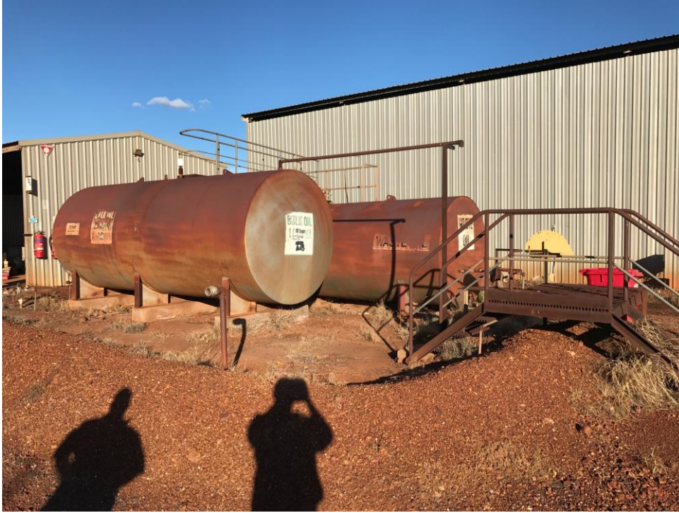
Figure 18 Bulk Oil / Waste Oil tanks.
